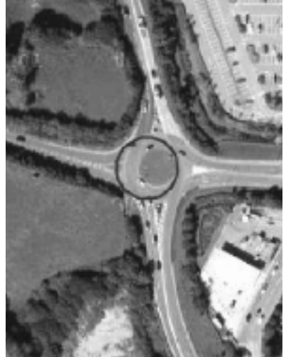
Work on the crossing at Kernick roundabout has been delayed
